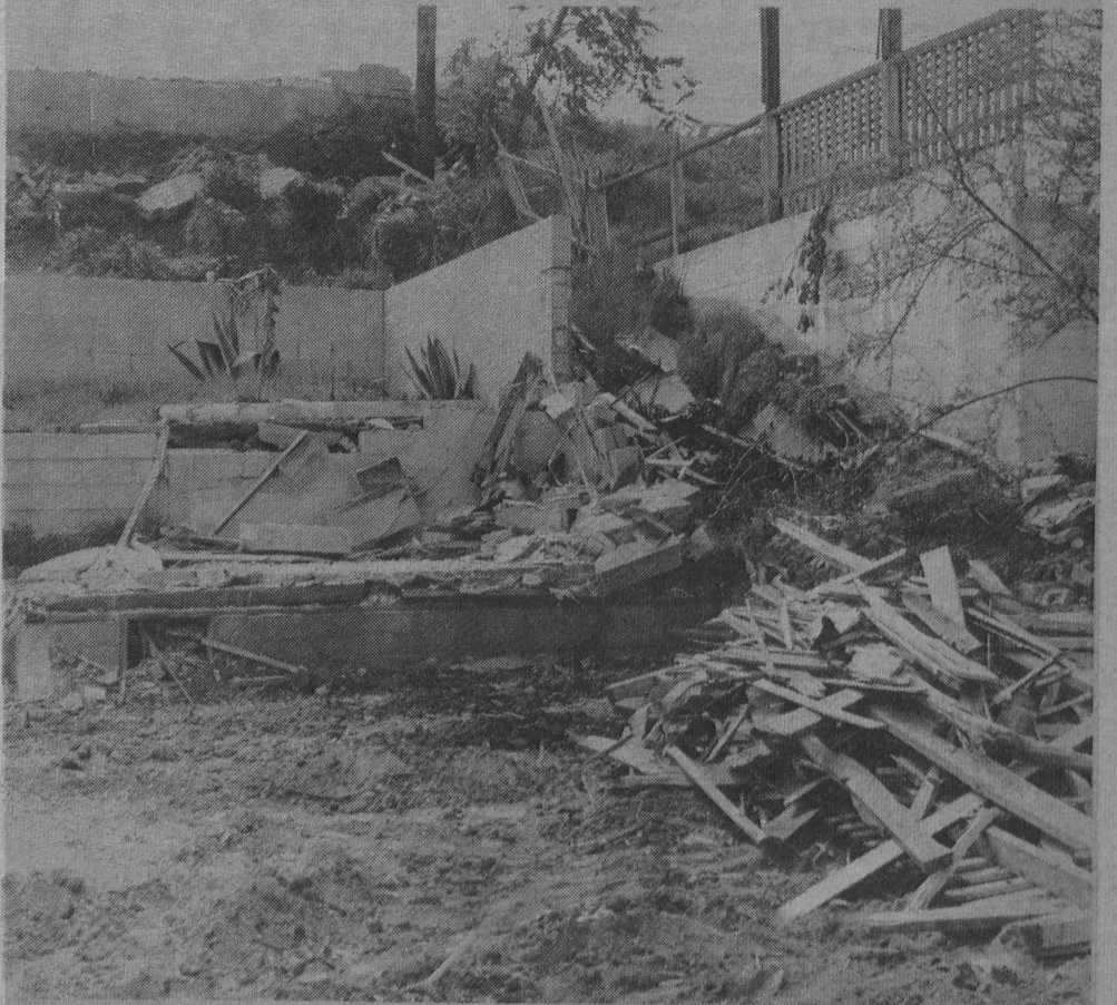
SOME WERE DESTROYED —Some of the houses near the school were torn down to make room for the expanding Cal State L.A. campus. The mix-master approach is cheaper for old houses that are not worth moving.
