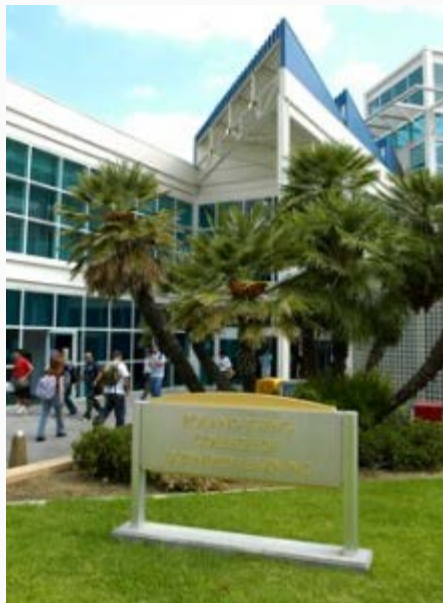
Tseng College building.
