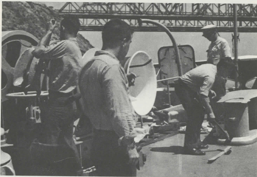
The Deck Men at Work
